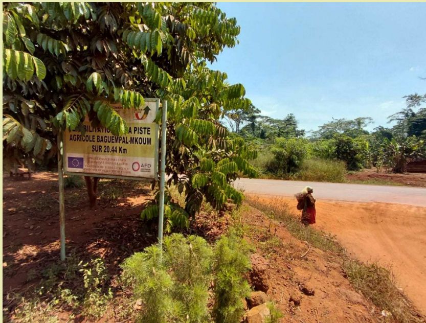
Picture 1 – On-the-spot visit to renovated rural access road
