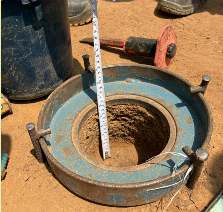
Picture 2 – On-site drilling test indicating discrepancies between actual road thickness and the technical specifications
