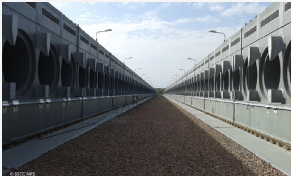
Picture 4: Dry spent fuel facility at Chernobyl
