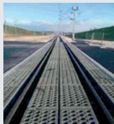
Photo 3 – New lines on the Perpignan-Figueras international section not yet used
