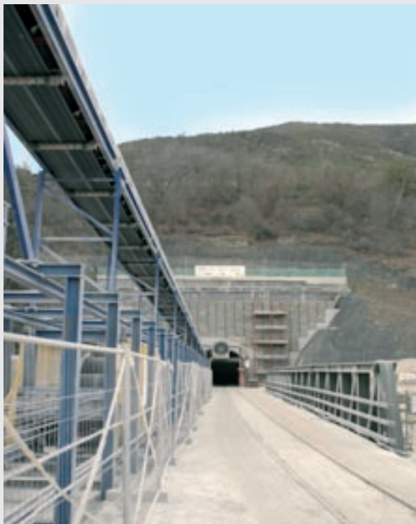
Photo 5 – Entrance to the exploratory tunnel for the Brenner Base Tunnel at Fortezza
