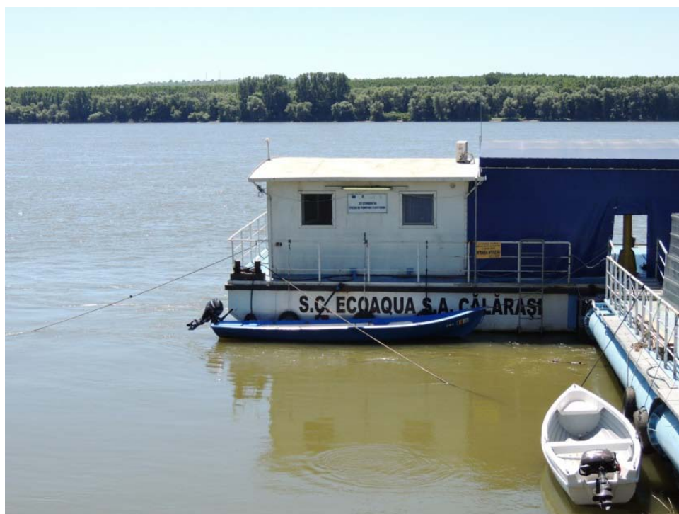
Picture 1 - Floating intake of water in Călăraşi (Romania)
