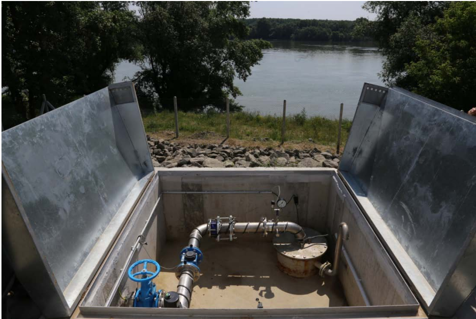
Picture 5 - Well providing bank filtered water from the Danube, Hungary
