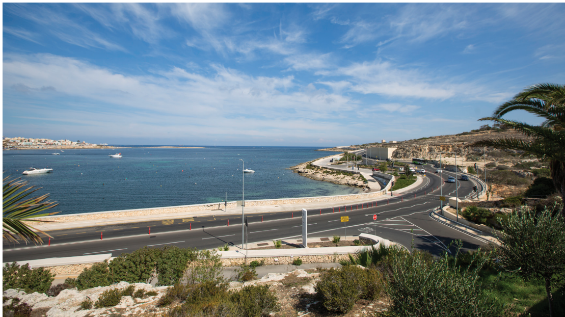
Upgrade Ten-T road Network, Malta
