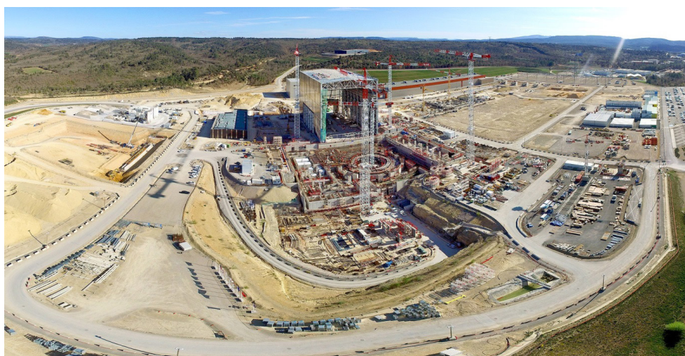
ITER work site-April 2016
