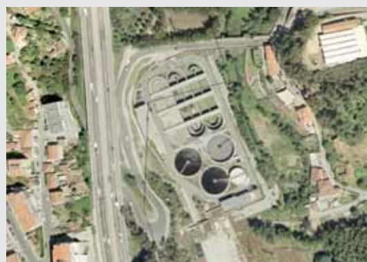
Picture 2: Febros treatment plant — Portugal
