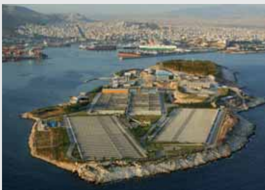
Picture 1: Psyttalia treatment plant — Greece
