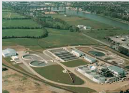
Picture 4: Drogheda treatment plant — Ireland
