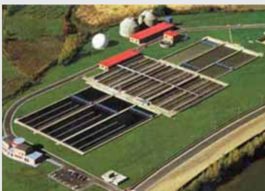
Picture 3: León treatment plant — Spain
