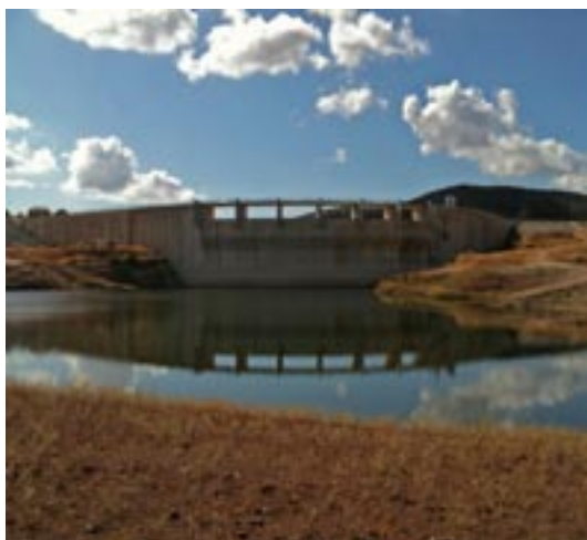
Picture 3: Dam in Spain
