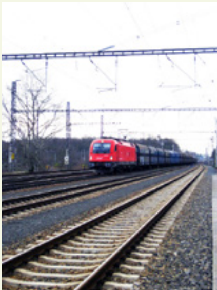
Photo 2 — A freight train passing through the reconstructed Břeclav railway junction (Czech Republic)
