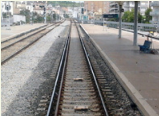
Photo 1 — Girona mercancías-Figueras bypass project (Spain)
